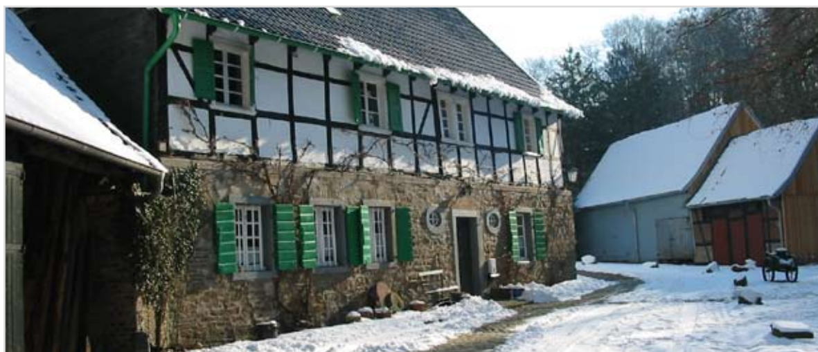
Figure 3: The historical Lamberts mill - a watermill, where decentralized waste water management is practiced. (Source: A. Rechenburg)
