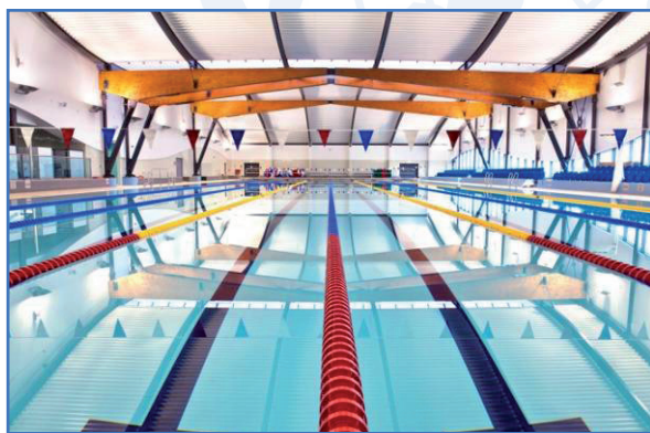
Figure1: View of an indoor swimming pool
