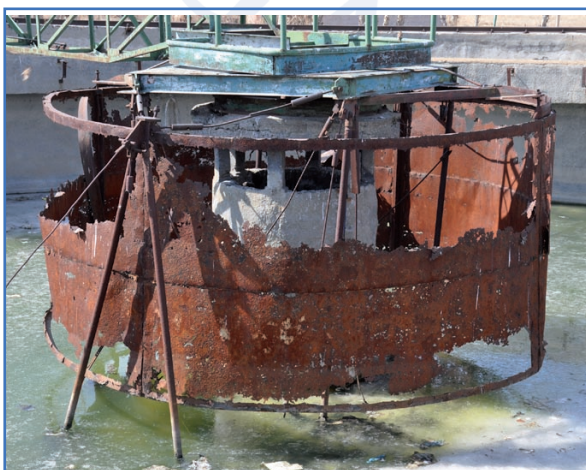
Figure 5: Central WWTP in Darkhan
