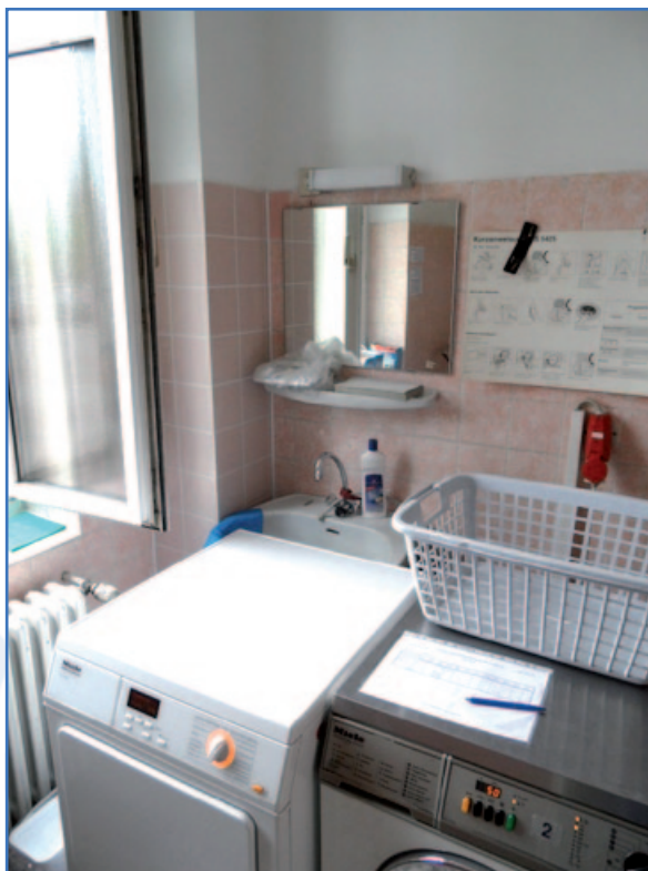
Figure 3: Poor accessible sampling point Source: IHPH
