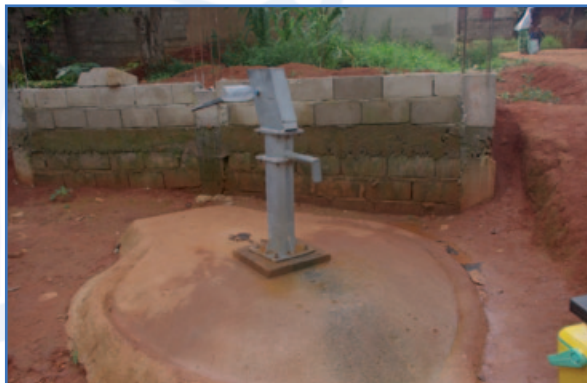
Figure 4: Well maintained dug well with a hand pump used by 400 people as drinking water supply Source: IHPH
