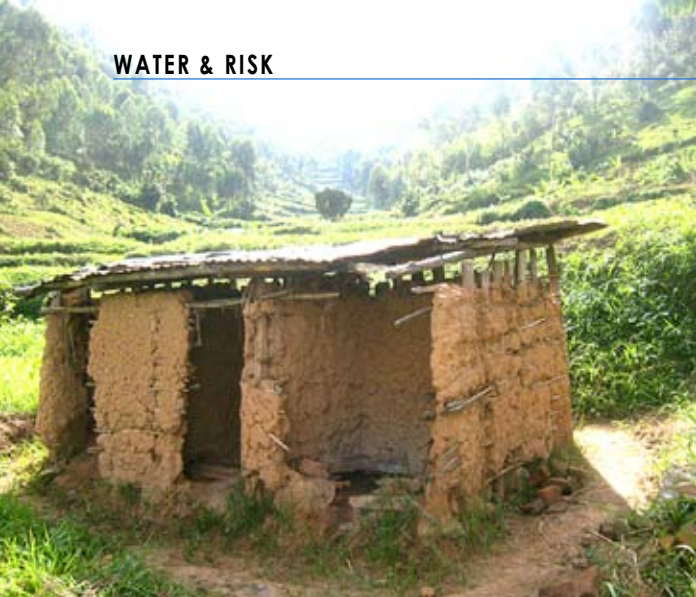
Figure 2: The old toilets Source: Claire Kwesiga
