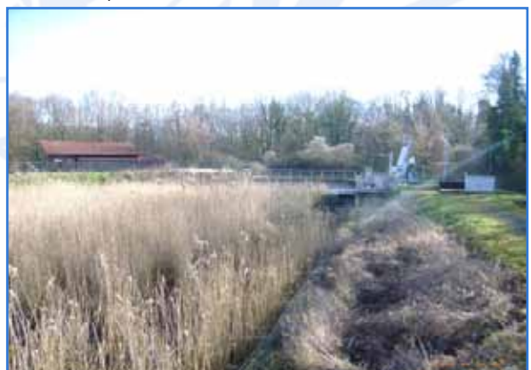
Figure 1: Retention soil filter (Source: Ertverband)
