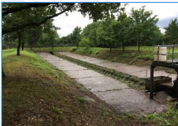
Figure 3: Sampling point for the analysis of stormwater discharge from a separation sewer system at the outlet of a rainwater retention basin (Source: Ertverband)
