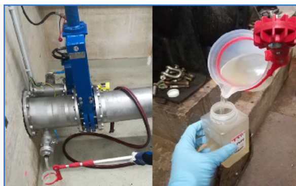
Figure 3: Wastewater samples taken at one of the sampling points within the wastewater system (Source: D. Schmiege)
